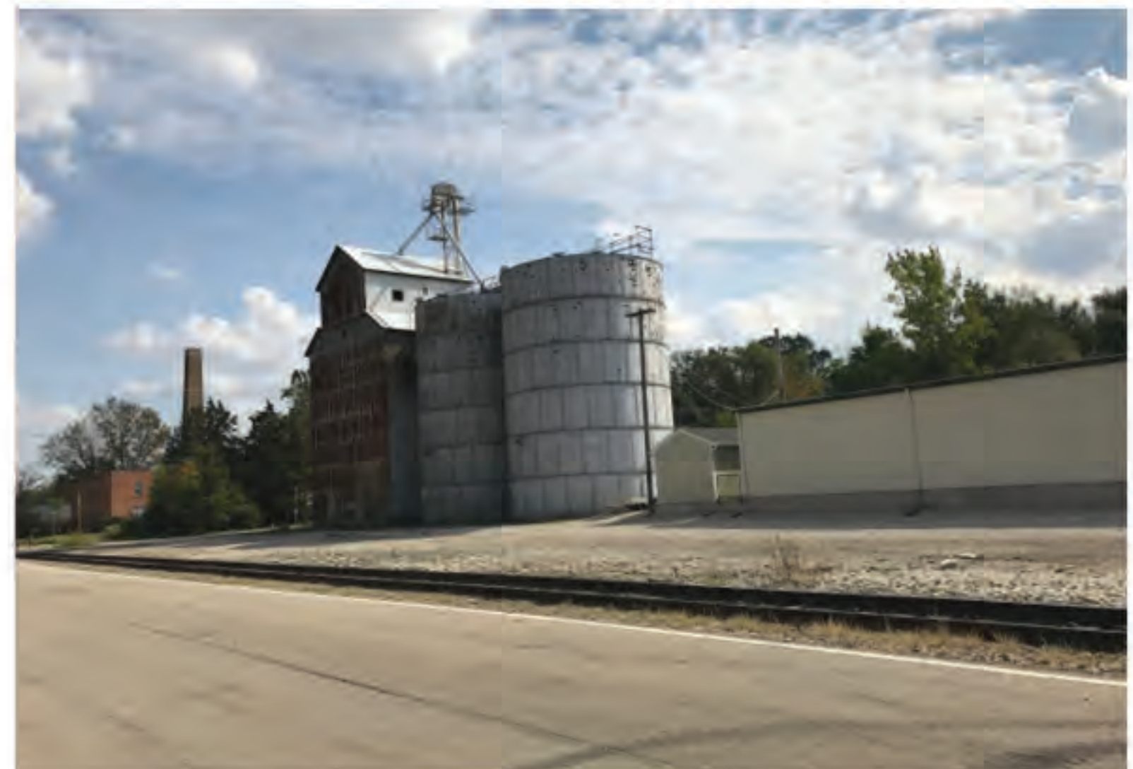
Figure X - Inactive Grain Elevator (Source)
