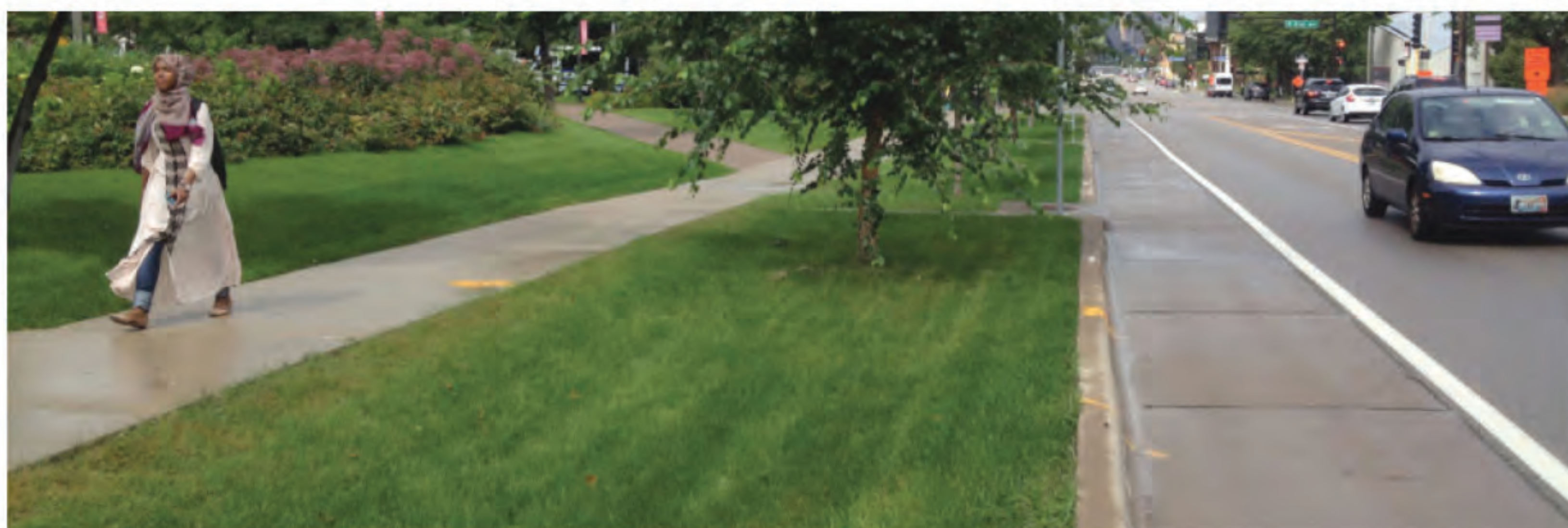
Figure X - Basic Roadside Swale (Source)
