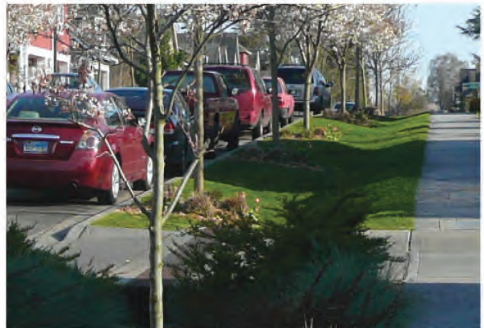
Figure X - Roadside Swale (Source)
