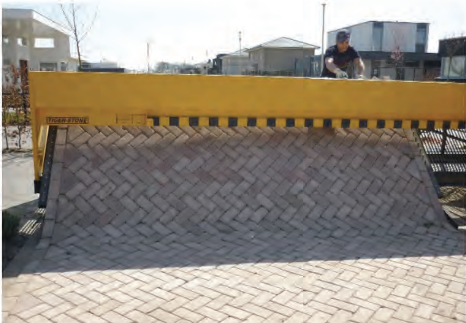
Figure X - Paver Laying Machine (Source)
