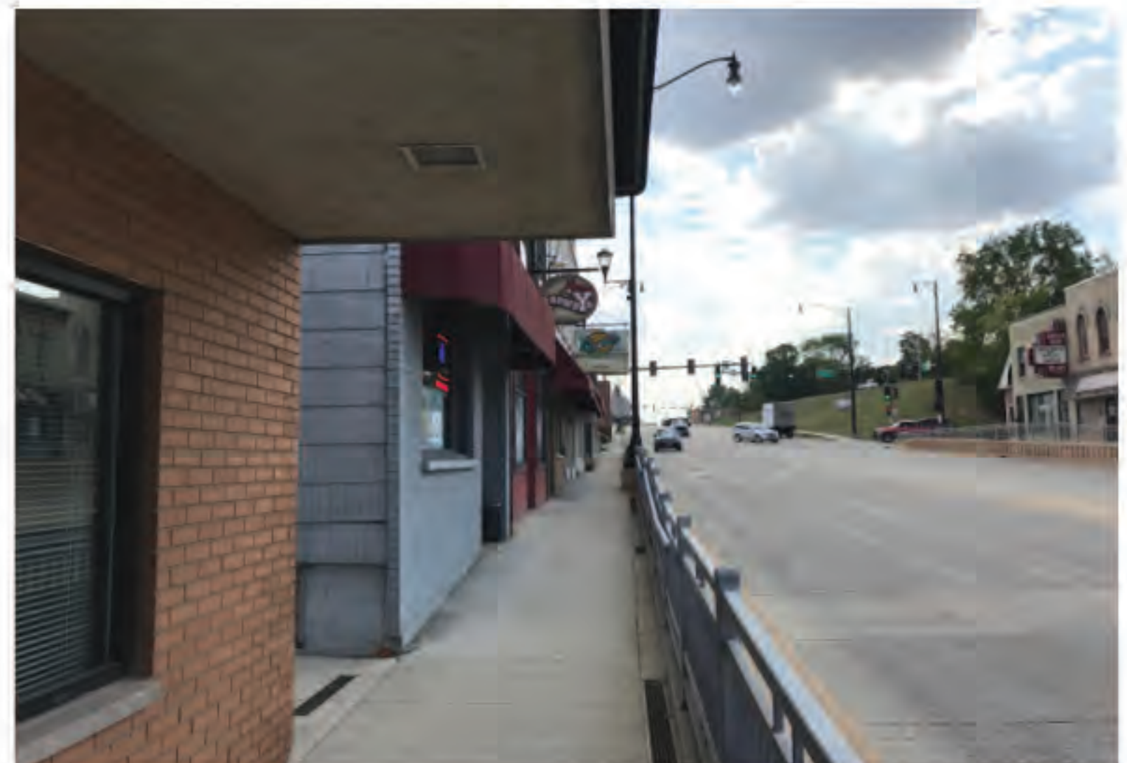
Figure X - Bridge Street Sidewalk and Barrier Wall (Source)
