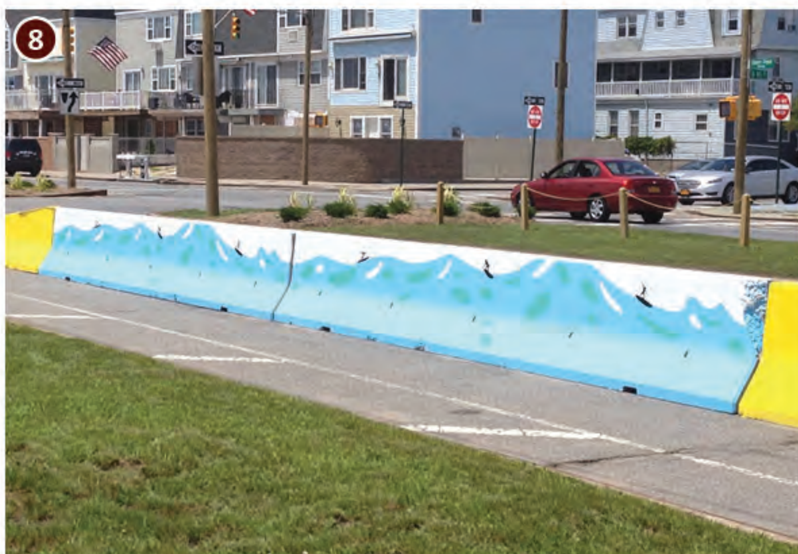
Figure X - Painted Concrete Barrier (Source)
