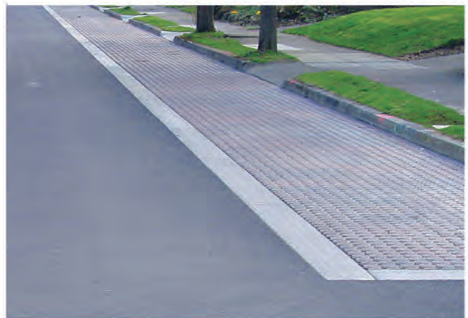
Figure X - Permeable Pavers for On-Street Parking (Source)
